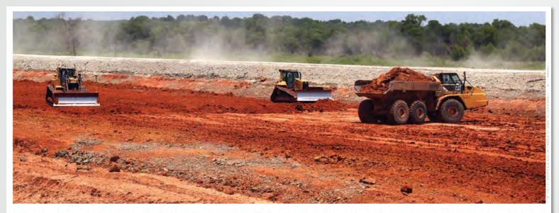
Contractors for the U.S. Army Corps of Engineers Tulsa District use heavy equipment to move tons of dirt while working on phase II of the Cumberland Levee Repair project along the Washita River, 12 miles east of Madill, Oklahoma. The levee was over-topped and breached June 21, 2015, during a record flood event brought on by historic amounts of rainfall across Oklahoma.
